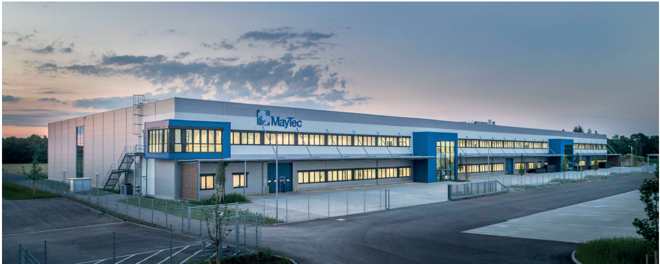
MayTec GmbH plant in Olching
